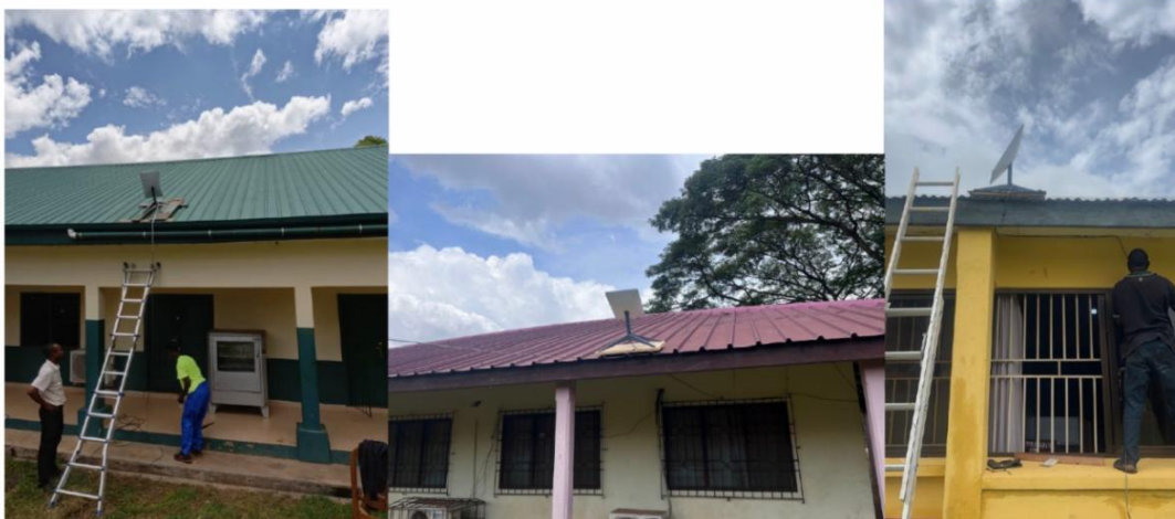
Starlink being installed at TVETs.
